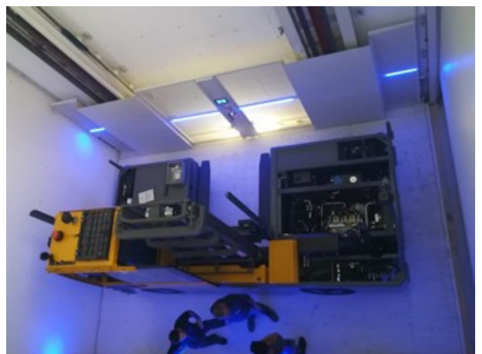
▼ Interior of a lifting platform.
